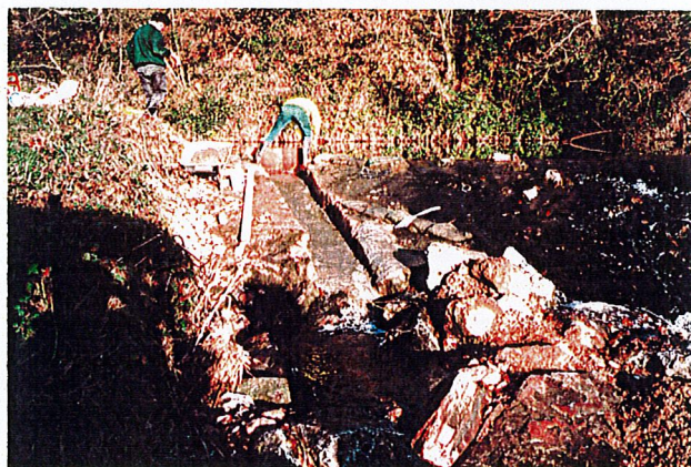
CUTTING THE NEW PATH UP OVER TIPTON WEIR
