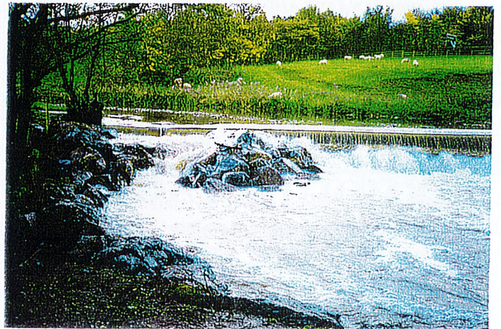
1997 IMPROVEMENTS AT TRACEY WEIR BY THE EA
