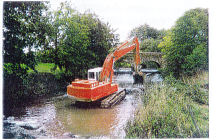
2001 LANGFORD WEIR A JOINT PROJECT WITH THE EA
