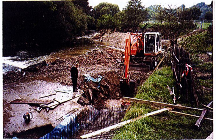
CONSTRUCTING OTTERTON FISH PASS
