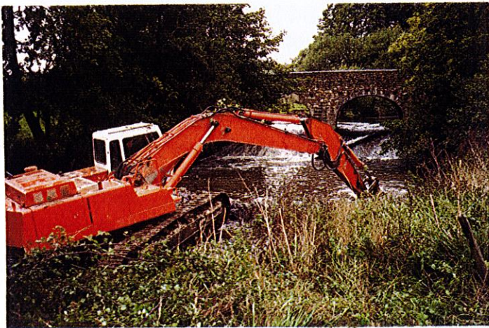
LANGFORD WEIR WORK IN PROGRESS
