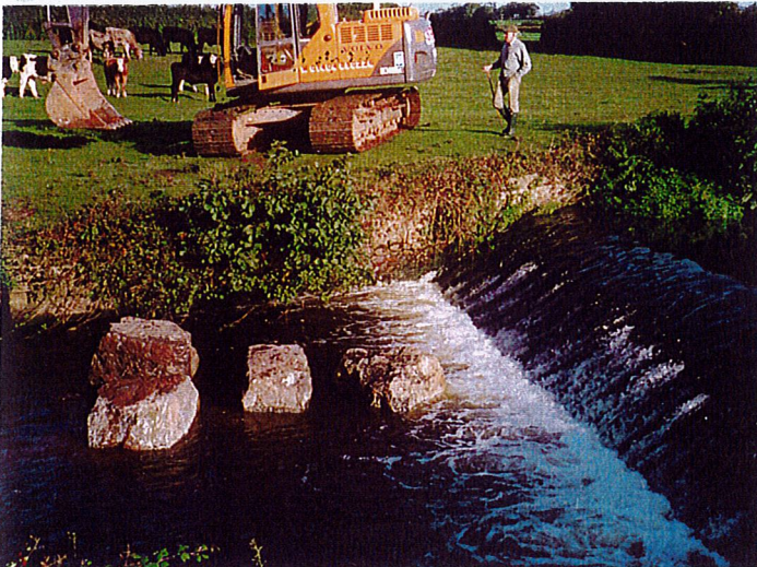
COLHAYES WEIR WORK IN PROGRESS
