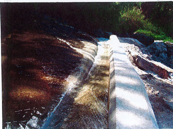
TIPTON WEIR NEW CHANNEL LHS PASS
