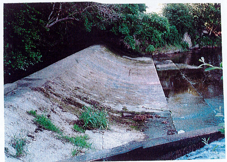
OTTERTON WEIR MAIN WEIR DRIED OUT 2005
