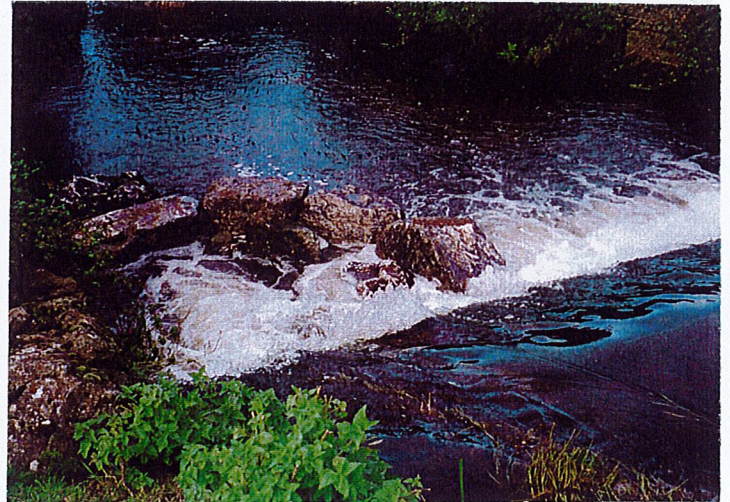
COLHAYES WEIR NEW SUB WEIR COMPLETED
